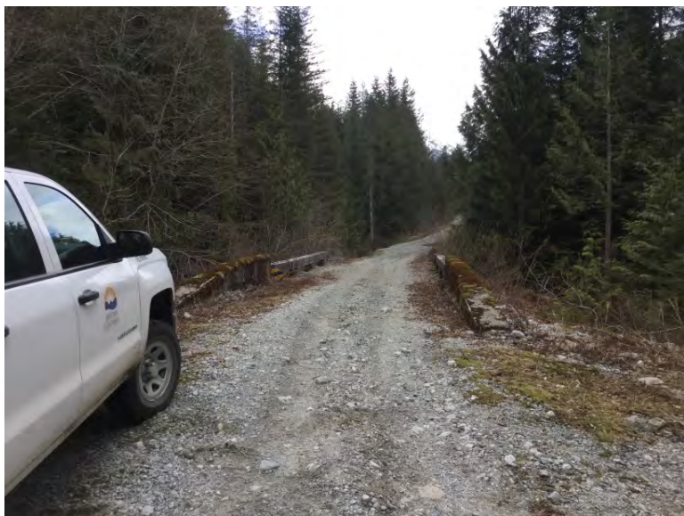
Approach from Right Bank when facing downstream
