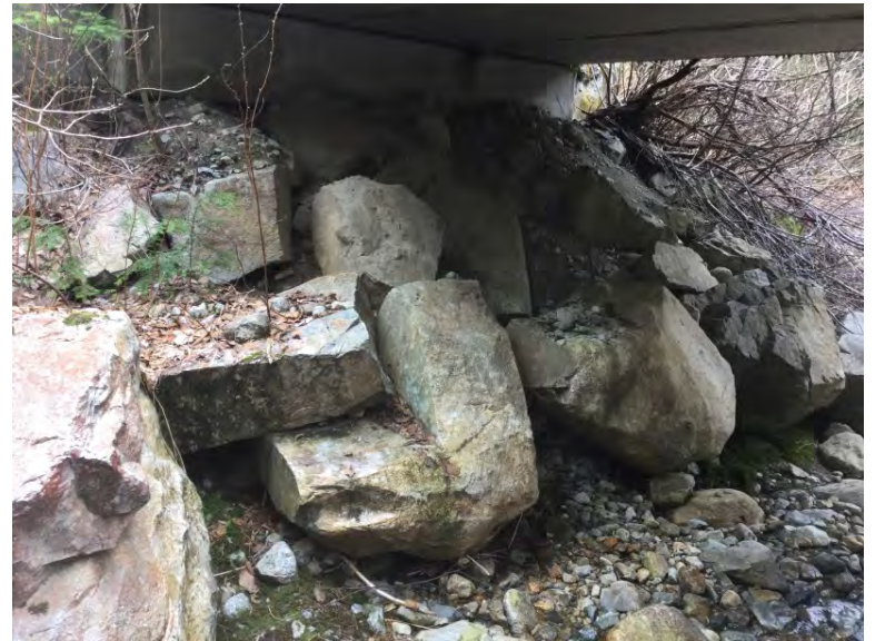
Left Bank Abutment when facing downstream
