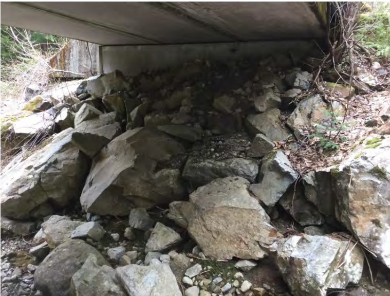
Right Bank Abutment when facing downstream
